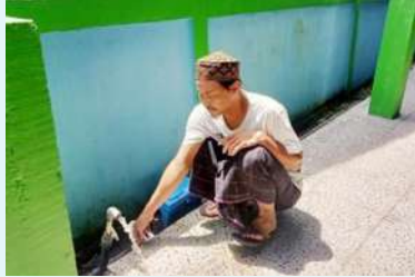
Penyaluran Supply Air untuk Kebutuhan MCK Masyarakat Setempat Pabrik Distribution of Water Supply for the Toilet Needs of Communities around the Factory [GRI 203-1] [OJK F.25]
